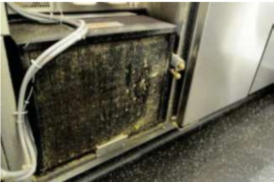
Blocked condenser coil
